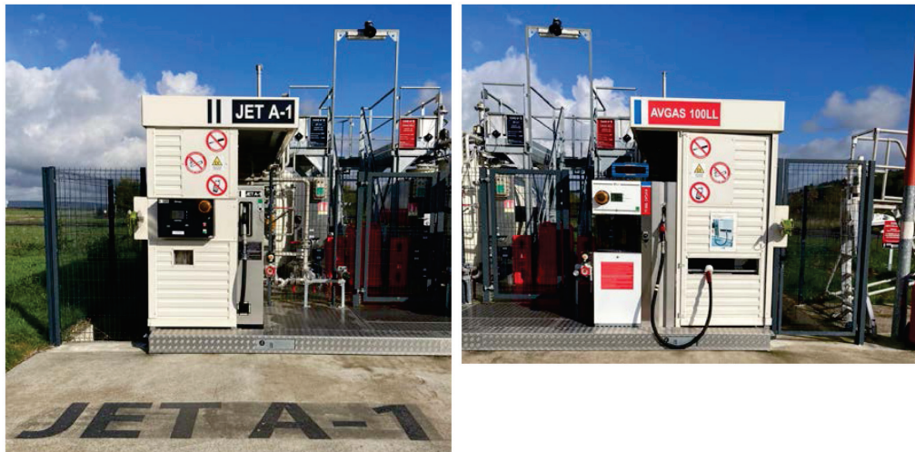
Figure 7a: Examples of fuel grade markings at stationary/fuelling trailer or kerbside fuelling cabinets
