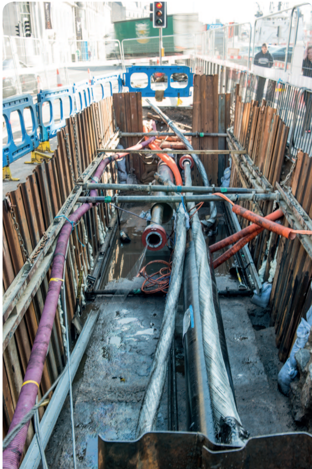
Jointing bay during construction showing temporary shuttering (Source: Balfour Beatty PLC)
