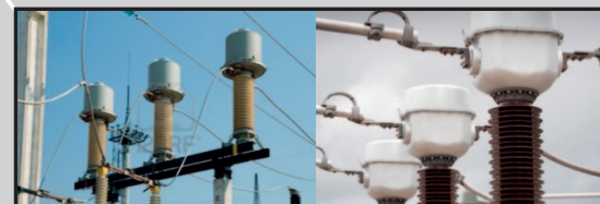
Measurement Transformers
