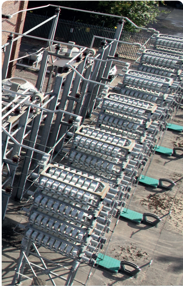
An example filter bank compound with static VAR compensation reactors (Source: National Grid)
