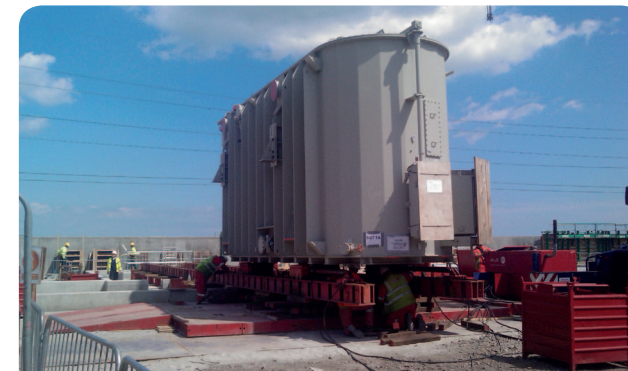
An example power transformer tank during installation (Source: Royal HaskoningDHV)
