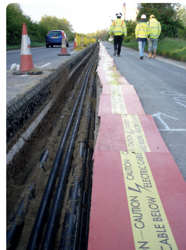
Cable ducting prior to trench infill (132kV) (Source: Royal HaskoningDHV)
