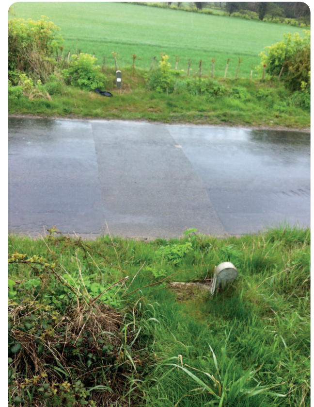
Image of buried cable route (road crossing) 1-2 years after construction (Source: Royal HaskoningDHV)
