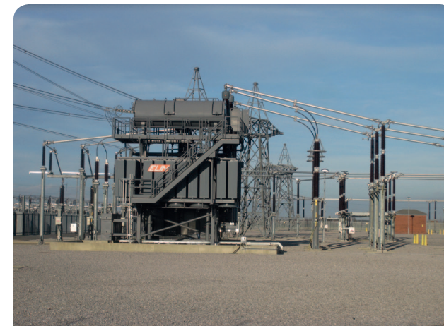
An example power transformer (Source: Royal HaskoningDHV)
