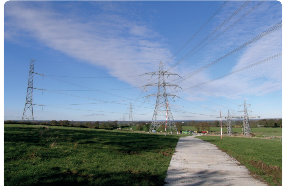
An example junction and corner tower (400kV) (Source: National Grid)
