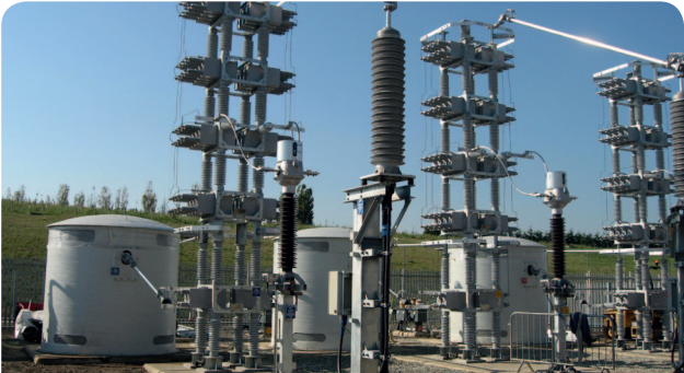
An example filter bank compound including reactors (in tanks) and capacitor banks (in racks) (Source: ABB Limited)
