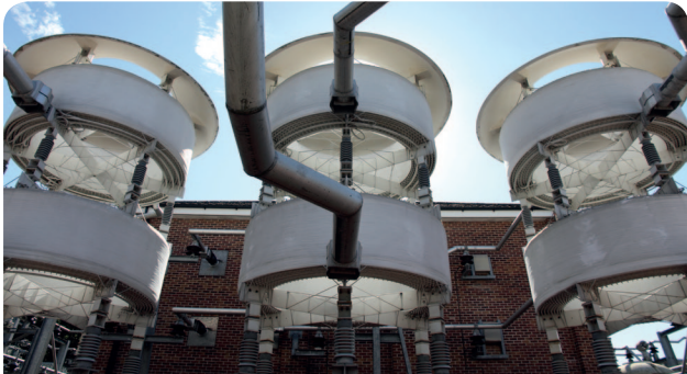
Static VAR compensation reactors providing reactive compensation (400kV) (Source: National Grid)
