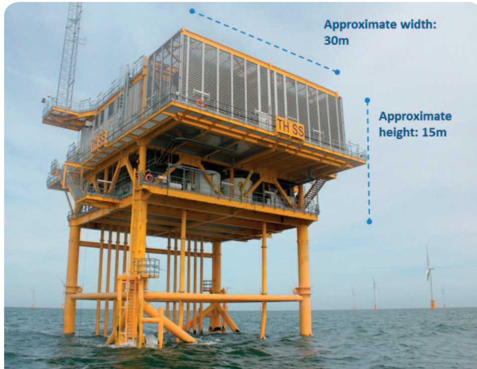
An example offshore AC substation (300MW) with jacket foundation - Thanet Offshore Wind Farm (Source: Royal HaskoningDHV)
