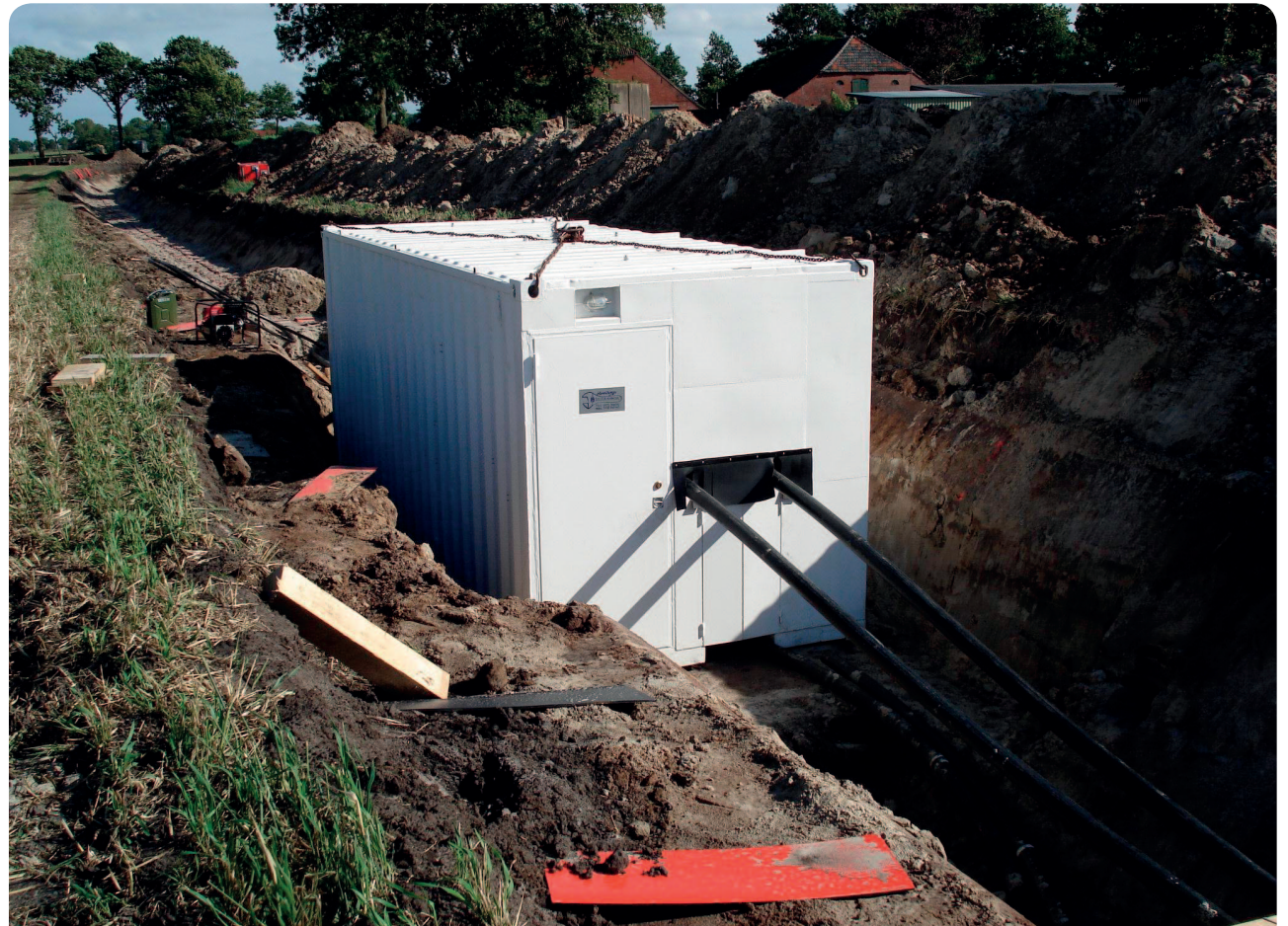
Temporary jointing container (Source: ABB Limited)
