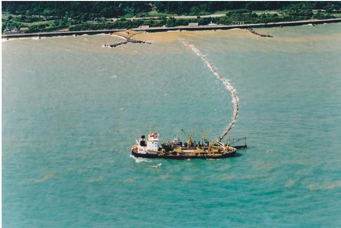
Figure 5.3 Vessel Engaged in Coastal Protection Works
