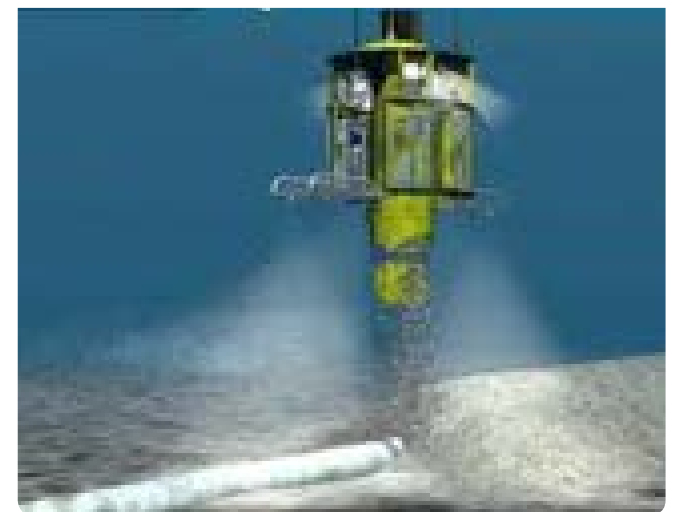
Figure 2-13 Fall-pipe application of a rock protection berm
