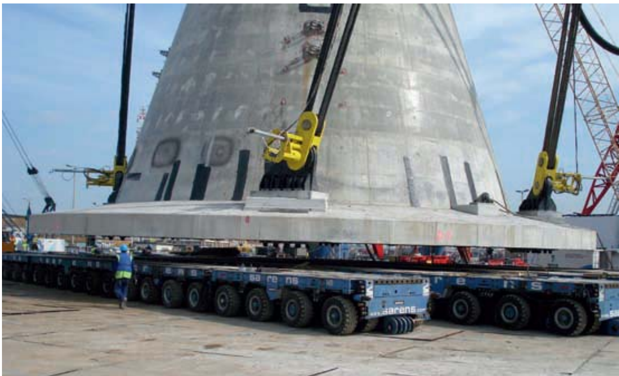
Figure 4-7 Gravity base foundation being prepared for lift-off from the quay (Source: Peire et al., 2009)
