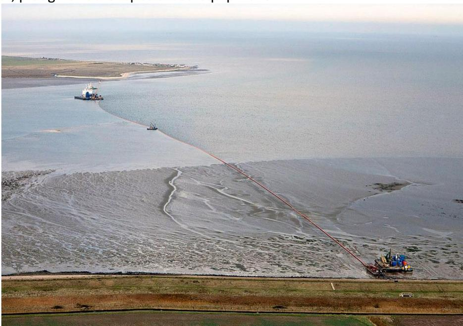
Figure 2: Illustration of shore pull during cable lay. Image courtesy of VBMS.
