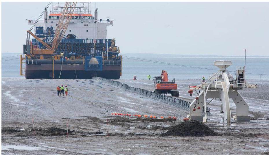
**Figure 4: Cable in position on a beach ready to start ploughing. The cable will be pulled from the vessel through the plough and anchored in preparation to start. Image courtesy of VBMS.**
