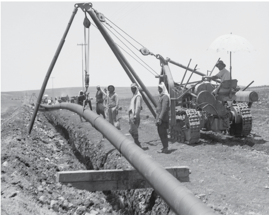
Dropping a welded pipe into a trench with a crane while laying the Iraq Petroleum Company's pipe line across Palestine's Plain of Esdraelon, July 1933. Completed in 1934 © Everett Historical - Shutterstock_244405399
