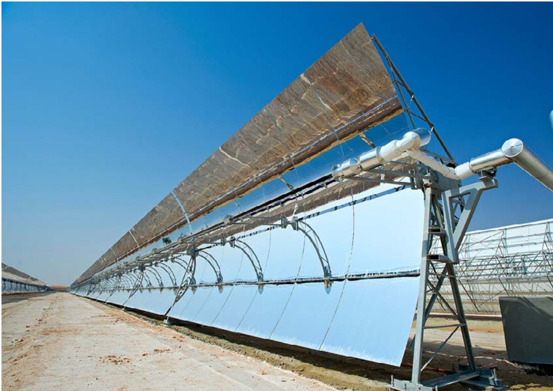
Shams 1 parabolic trough in Abu Dhabi © Masdar Official https://www.flickr.com
