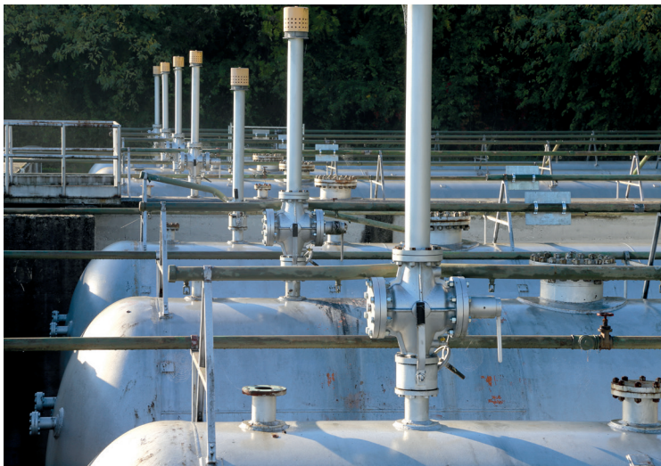
Pressurised tanks for storing methane at a refinery
