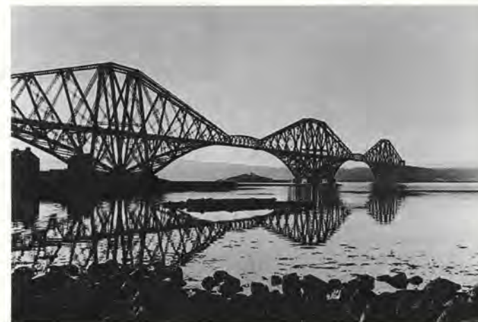
The 100-year old Forth Bridge.
