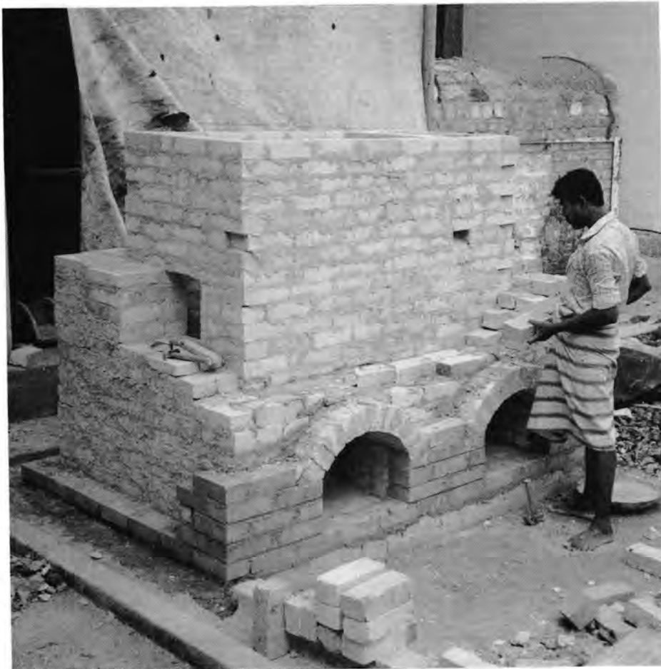
Constructing the rice husk furnace in Sri Lanka.
