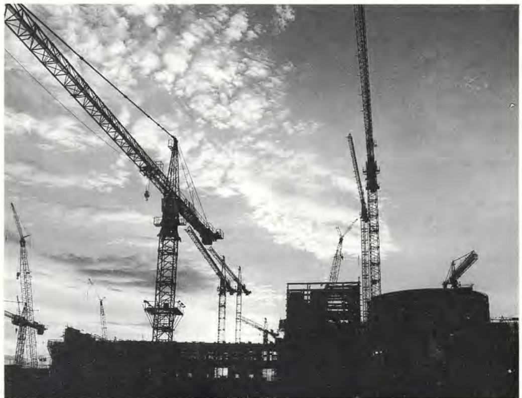
Sizewell B under construction.
