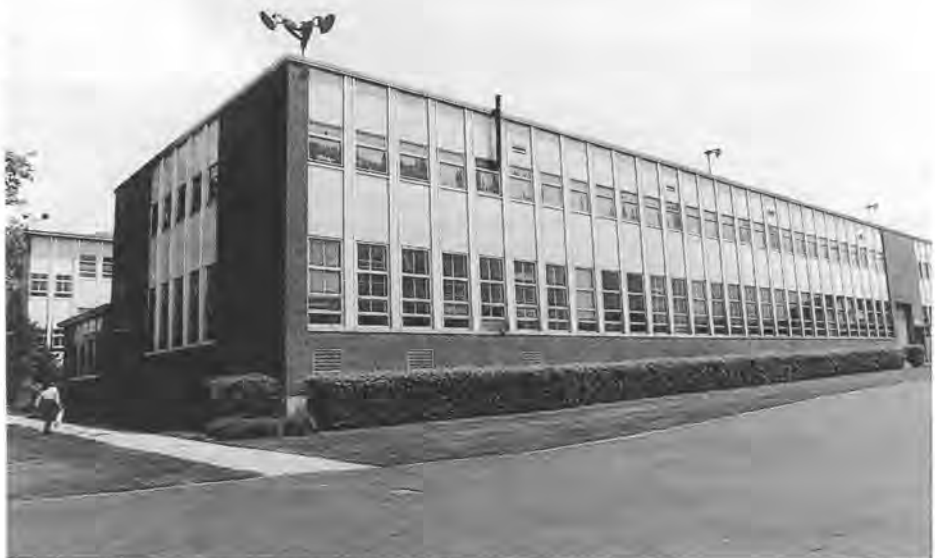
The Westinghouse pre-pilot manufacturing facility.
