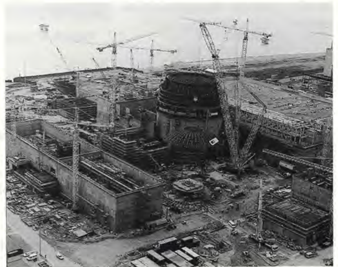
Figures 5 and 6: Left, aerial view of the site in May 1991. Right, shows the hemispherical dome and the Gottwald crane.
