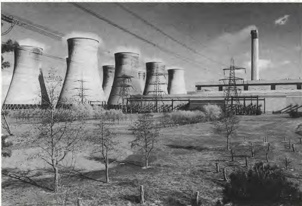
National Power's Eggborough power station.
