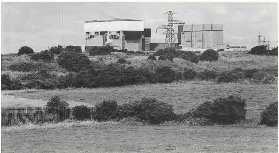
Nuclear Electric's Heysham 1 and 2 power stations.
