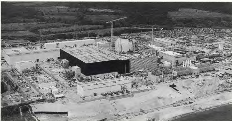
Figure 7: aerial view of the site in July 1992.
