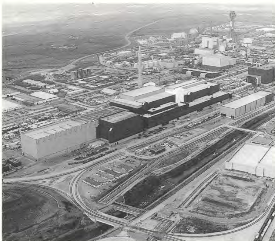
Aerial view of THORP, receipt and storage facility and pond extension.
