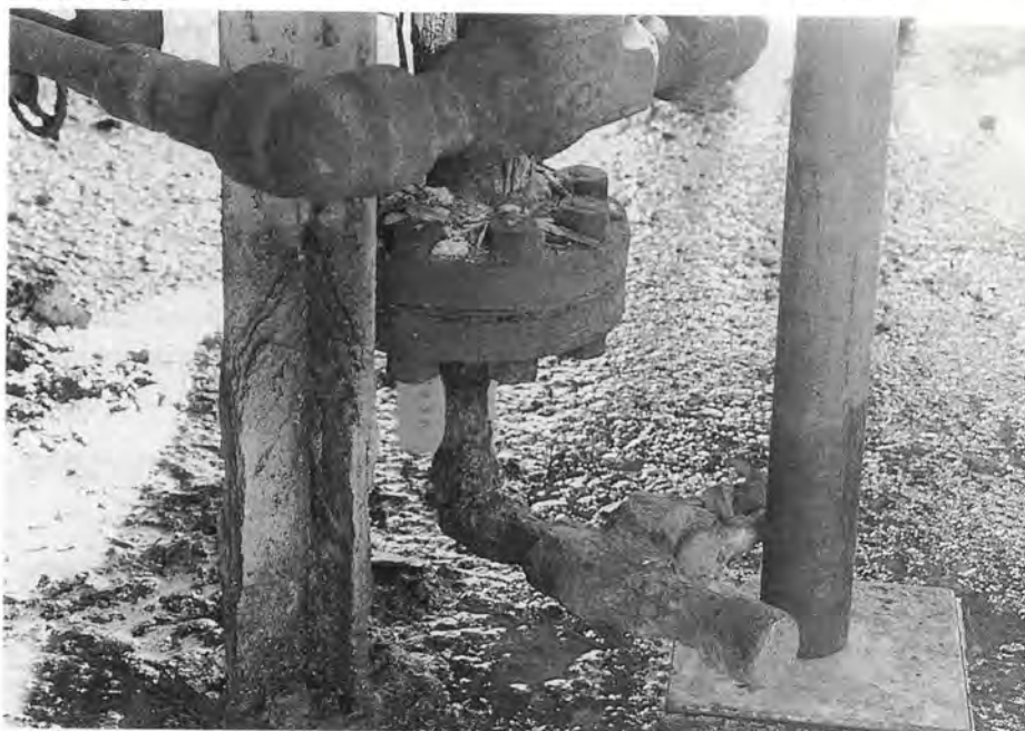
The compound forms a new seal, stopping the leak.
