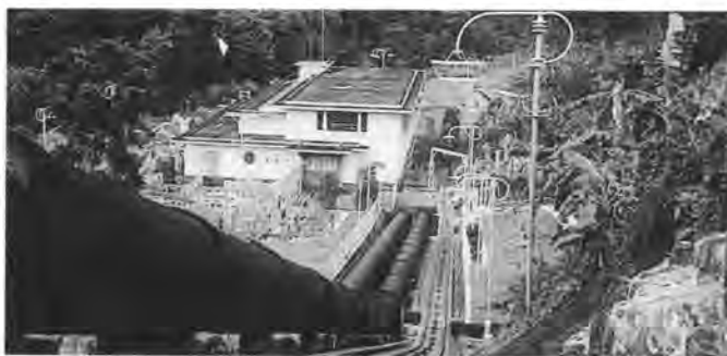
A comprehensive investment programme by the state authority of Java includes the modernisation of seven of the Island's hydroelectric plants, such as the one above left. The programme order has gone to Sulzer-Escher Wyss, who estimate that the modernisation should increase output by 20 630 kW to a total of 92 980 kW, and ensure safe, cost-effective operation for the next 25 years. Computer-aided runner design methods (above right) will be used in revamping the old power stations.
