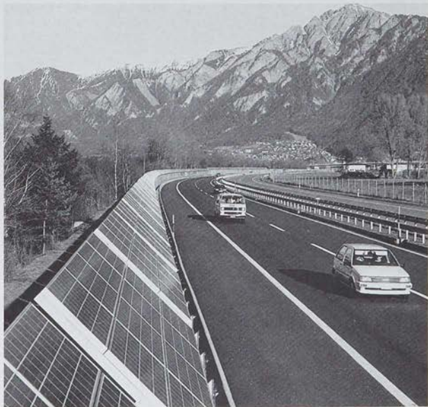
Solar panels on the N13 motorway in Switzerland, part of their photovoltaic programme.
