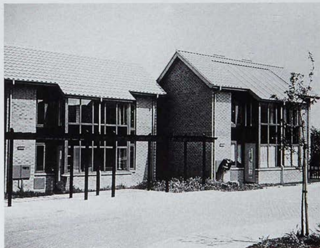
Houses in Milton Keynes with, on the right, a roof-space collector, and on the left without. Both have most of the windows on the south side.
