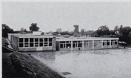
Nazeing County Primary School in Essex, left prior to refurbishment. This was a typical system-built school in urgent need of improvements in the weatherproofing and thermal performance of the building fabric. Right, the school after refurbishment. Thermosyphoning air panels providing solar heated air were incorporated as part of the curtain walls. They can be seen as the opaque elements which alternate with pairs of windows.
