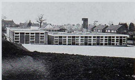
Nazeing County Primary School in Essex, left prior to refurbishment. This was a typical system-built school in urgent need of improvements in the weatherproofing and thermal performance of the building fabric. Right, the school after refurbishment. Thermosyphoning air panels providing solar heated air were incorporated as part of the curtain walls. They can be seen as the opaque elements which alternate with pairs of windows.
