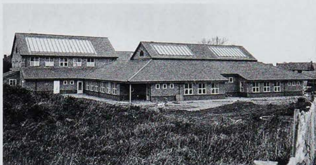
Green Park School, Newton Pagnell, showing roof space collectors for preheating air before it enters a gas-fired warm air heating system.
