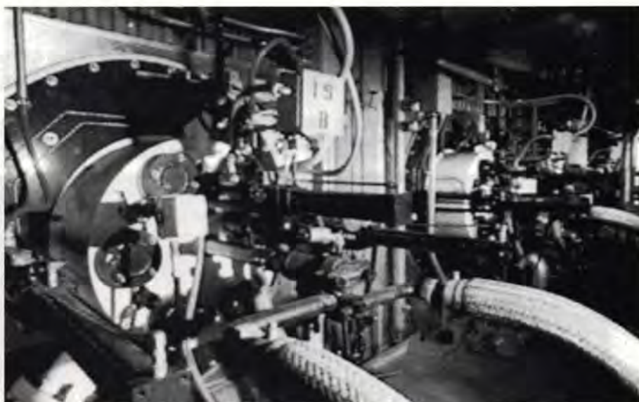
Todd Dynaswirl-LN burners on two 750 MW supercritical Foster Wheeler boilers located in Southern California
