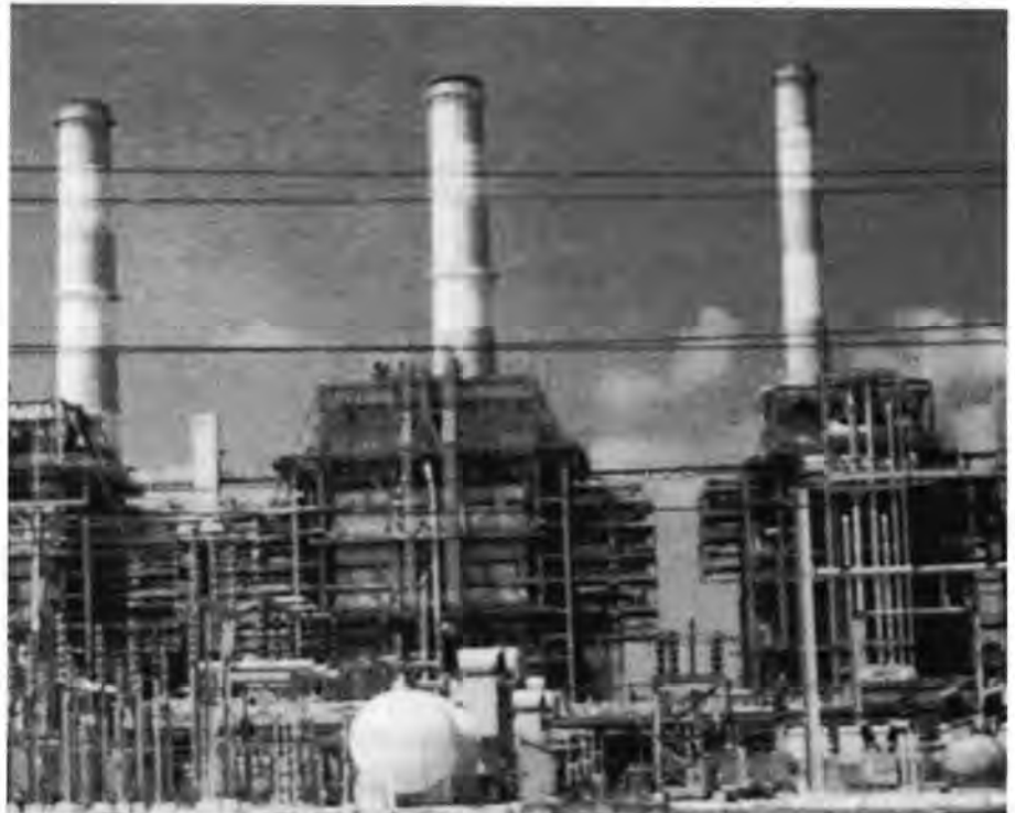
Two 400 MW gas/oil fired utility boilers being retrofitted with 36 Todd Dynaswirl-LN low NO x burners at a Florida utility.
