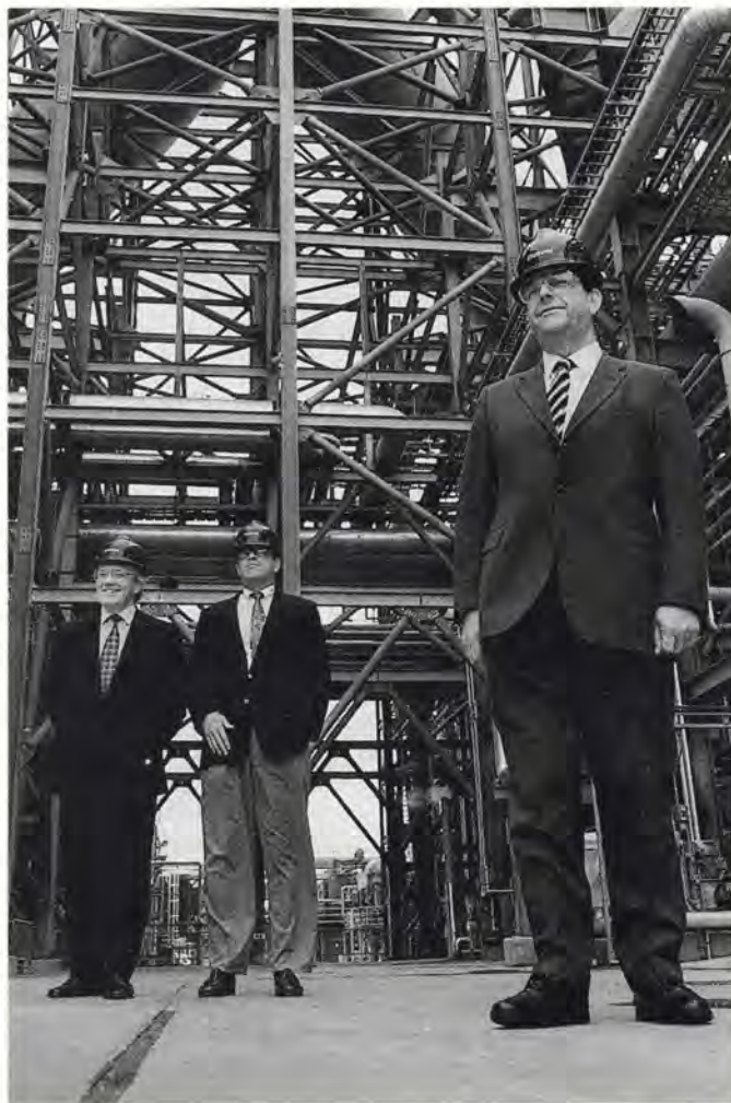
September saw the official opening of the Central Area Transmission System (CATS) and Teeside power station by Lord Wakeham (above, right). The project marks the first time North Sea gas has been piped ashore directly to a major industrial area in the UK. The 250-mile CATS pipeline comes ashore at Coatham Sands and then crosses under the Tees to the Seal Sands site. The project is a joint venture between Amoco, Amerada Hess, British Gas, Phillips, Agip and Fina. Close to 300 million cubic feet of gas per day will provide fuel for Teeside power station on a 15-year contract. Teeside is the world's largest gas-fired combined heat and power plant at 1875 MW, and began commercial operation in April this year. Its process steam goes to nearby ICI.
