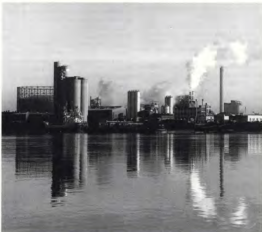
Tunnel Refineries at Greenwich in south east London was one of the first process manufacturers in the UK to recognise the tremendous advantages of combined heat and power. Their 15 MW CHP plant was commissioned in October 1990.
