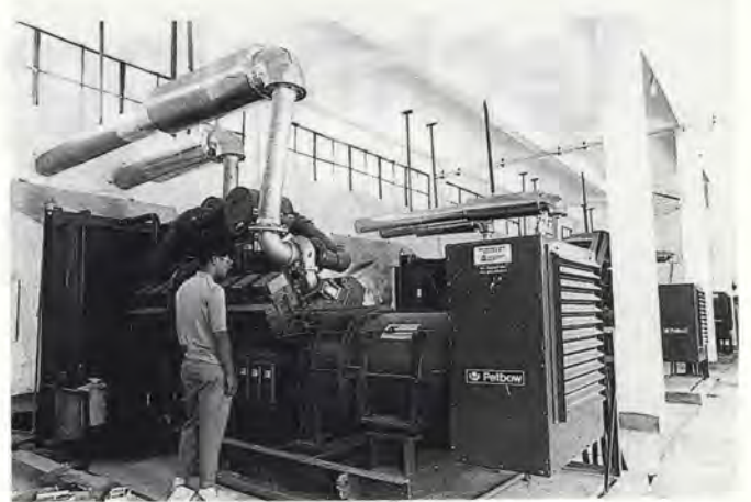
A 4MW power station has been installed in the Chinese municipality of Baoan in Lung Gang, Guangdong Province to provide essential baseload operation for the region's power supply bureau of local government. The area has been designated an important production area, needing a continuous, reliable power supply — both for existing factories and to attract new businesses.
