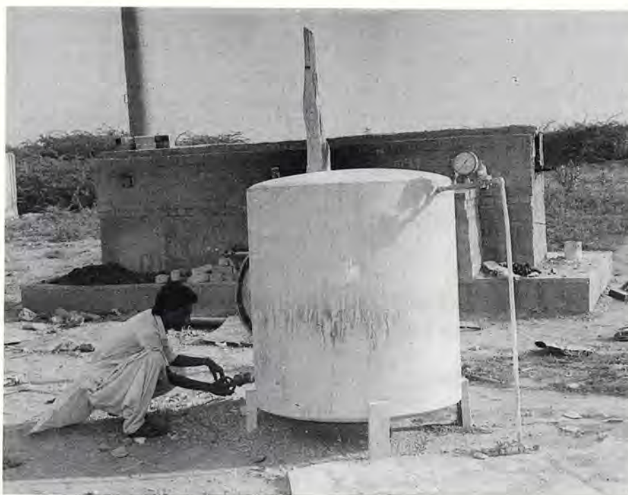
An Indian design of biogas plant.
