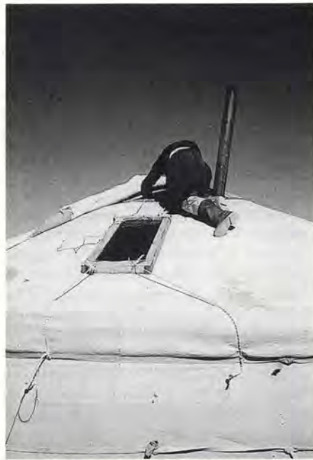
An 11 W peak, Chinese manufactured solar PV module and lighting system being installed on a nomad's tent (ger). Total installation time was a mere 90 seconds!
