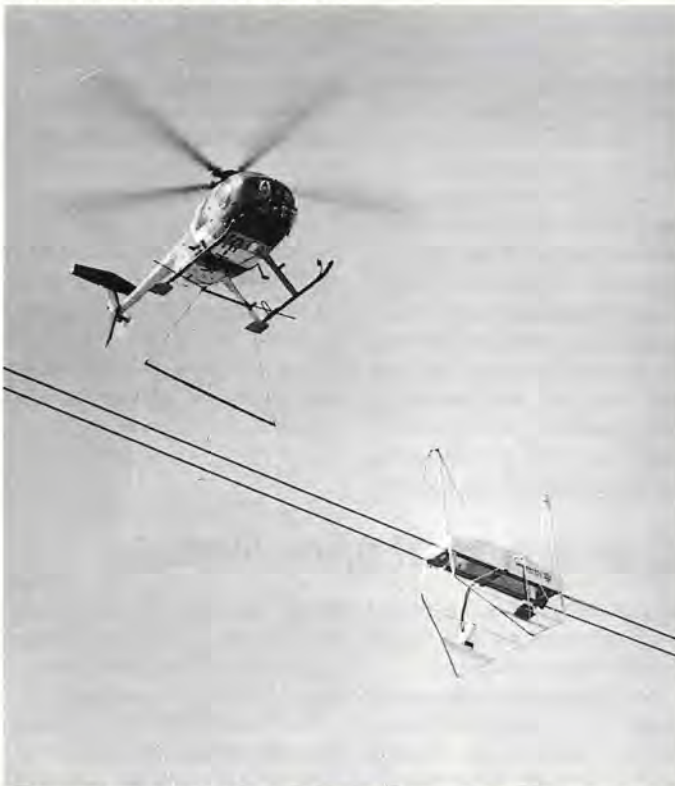
A new Swedish robot device controlled from a helicopter can check and repair power lines, without taking the line out of service. Dubbed 'Robhot' (robot for hotline works), the device has been developed by Swedish power transmission company Vattenfall Transmission AB, who has submitted a patent application. Of particular use for checking splices, the robot is lowered from the helicopter on a kevlar line. A fibre-optic link to the helicopter carries all the control and measurement signals, carrying out the work in a fraction of the time taken by conventional methods.
