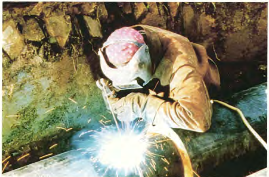
Installation of highly insulated heat distribution pipes.
