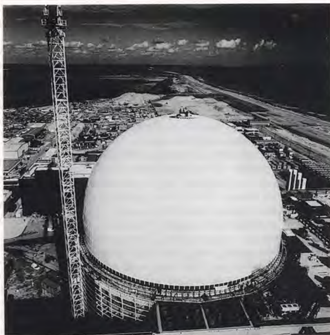
Fixing the cladding to the secondary containment dome at Sizewell B involved the use of one of the tallest tower cranes in the UK. Roofers had to work in specially-designed cradles. "The project called for some highly original thinking" said David Parnell of E H Smith (Roofing) Ltd.
