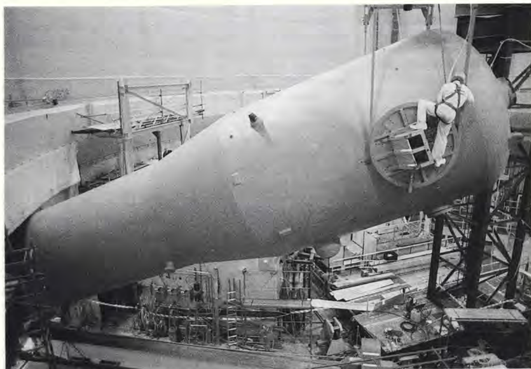
At Beznau 1 nuclear power plant, near Zurich, Switzerland, the two steam generators were replaced with the precision of a watchmaker. The main activities in the reactor building were completed in just 44 days, during which time it was also possible to replace sections of the reactor coolant line. The contract was awarded to the power generation group of Siemens AG in consortium with Sulzer Thermtec AG. The picture shows one of the new steam generators, weighing around 205 tonnes, being rigged into position.
