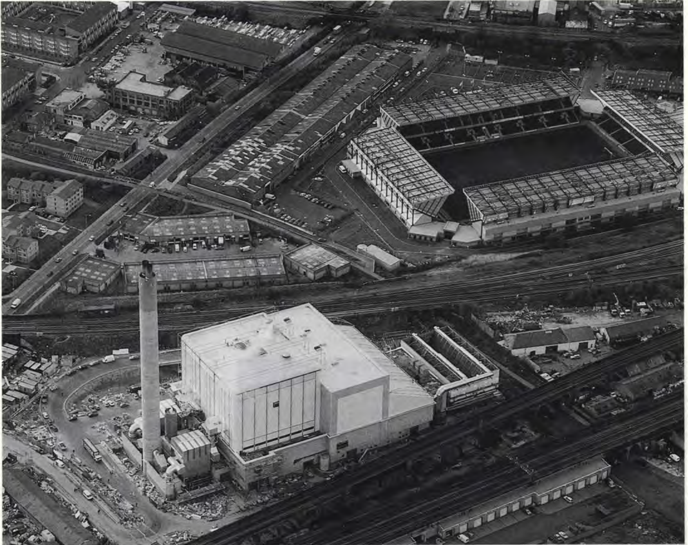
The SELCHP plant at Deptford in London. Millwall football ground is situated top right of the picture, with the access route for the lorries carrying municipal waste on the bottom left.
