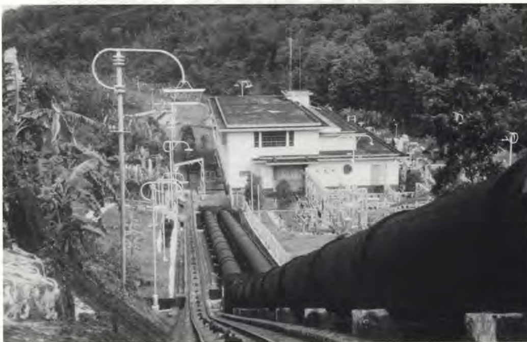
With the recommissioning of the last of a total of 22 turbines, Sulzer Hydro recently completed its largest renovation contract in South-East Asia. It entailed the renovation of seven hydropower plants on the island of Java, Indonesia, and was valued at 25 million CHF. As a consequence of the renovation, Sulzer was able to increase the output of the turbines, which in some cases were up to 60 years old, by 10 to 20%, and to ensure the economics and safety of the plants for a further 25 years. The project supports the go-ahead industry, inasmuch that it fulfils its requirement for reasonably priced energy. The picture shows Jelok, one of the seven hydropower plants.
