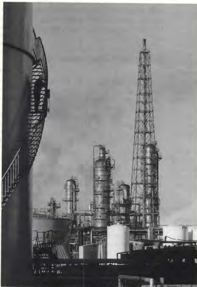
Leading UK manufacturer and exporter of chemical products, BASF plc, has signed a 15-year contract with National Power to buy electricity and steam from a new CHP plant. The £32 million plant will be integrated into the existing steam raising plant at BASF's 300 acre complex at Seal Sands on Teeside.
