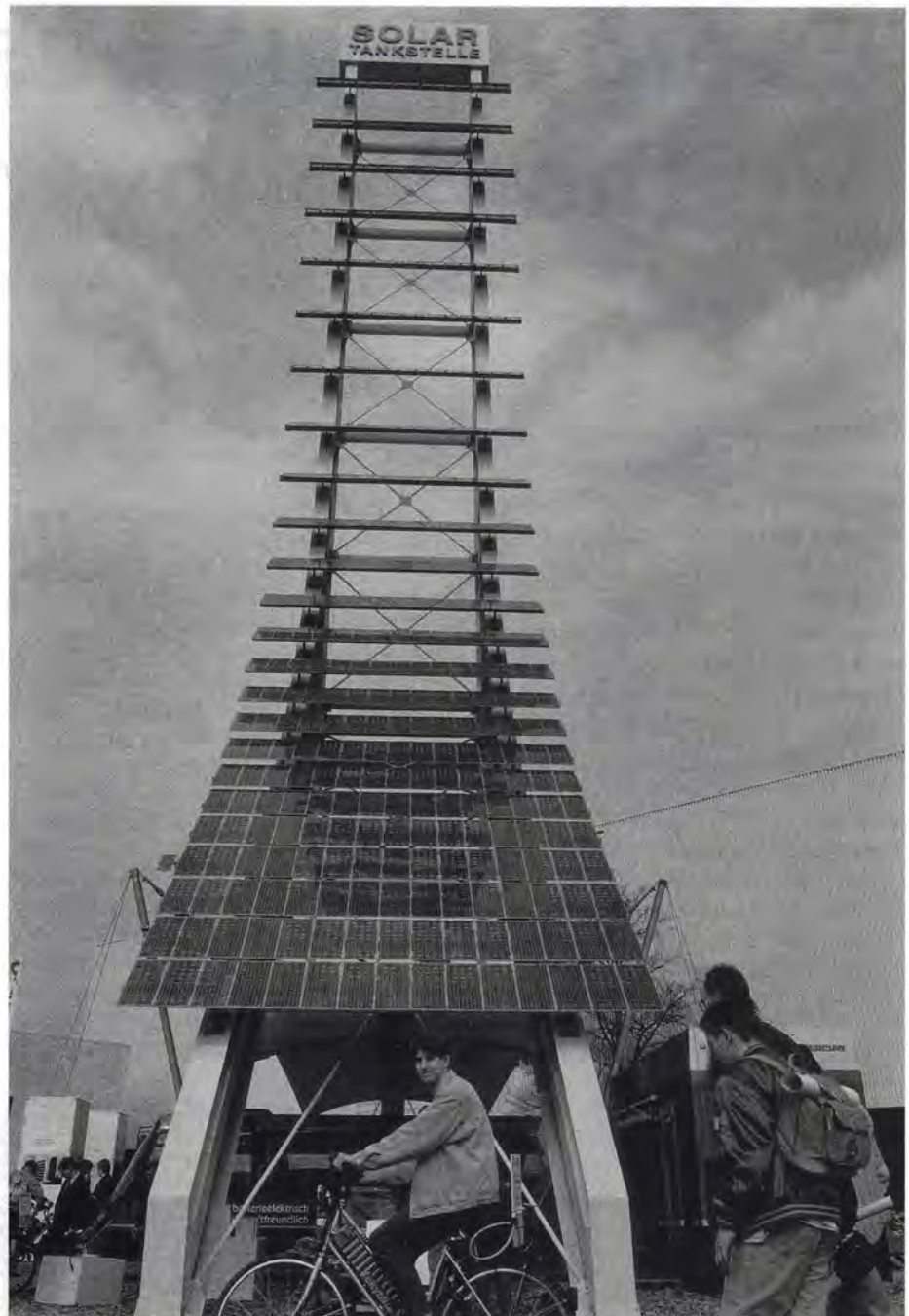
PHOTOGRAPH COURTESY OF DEUTSCHE MESSE AG The solar tankstelle, 42.5 meters high, with a maximum output of 15 kW.
