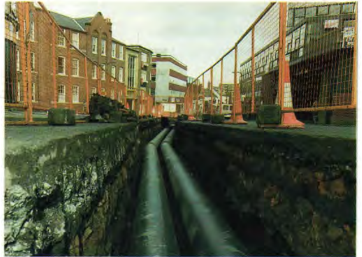
Pipework installation—the insulated heating mains are installed underground
