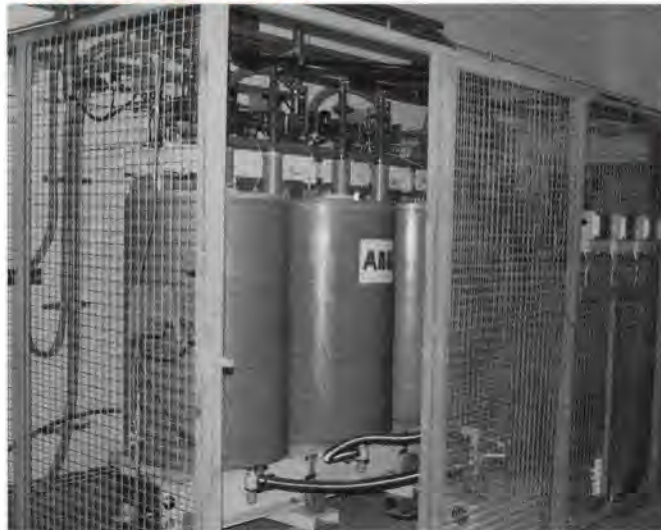
The high temperature superconducting distribution transformer connected to the Swiss electricity grid.
