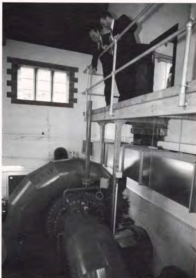
Ron Davies, Secretary of State for Wales (left), at the opening of Britain's latest green power station - a 4.2 MW hydro-electric project at the Elan valley, near Rhayader in mid Wales. Built by Hyder Industrial, the £5.2 million project comprises five small hydropower stations at the foot of the valley's four dams.
