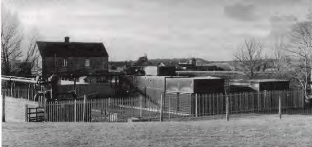
Haul Waste's landfill gas-to-energy site in Ardley, Oxfordshire uses one Caterpillar engine
