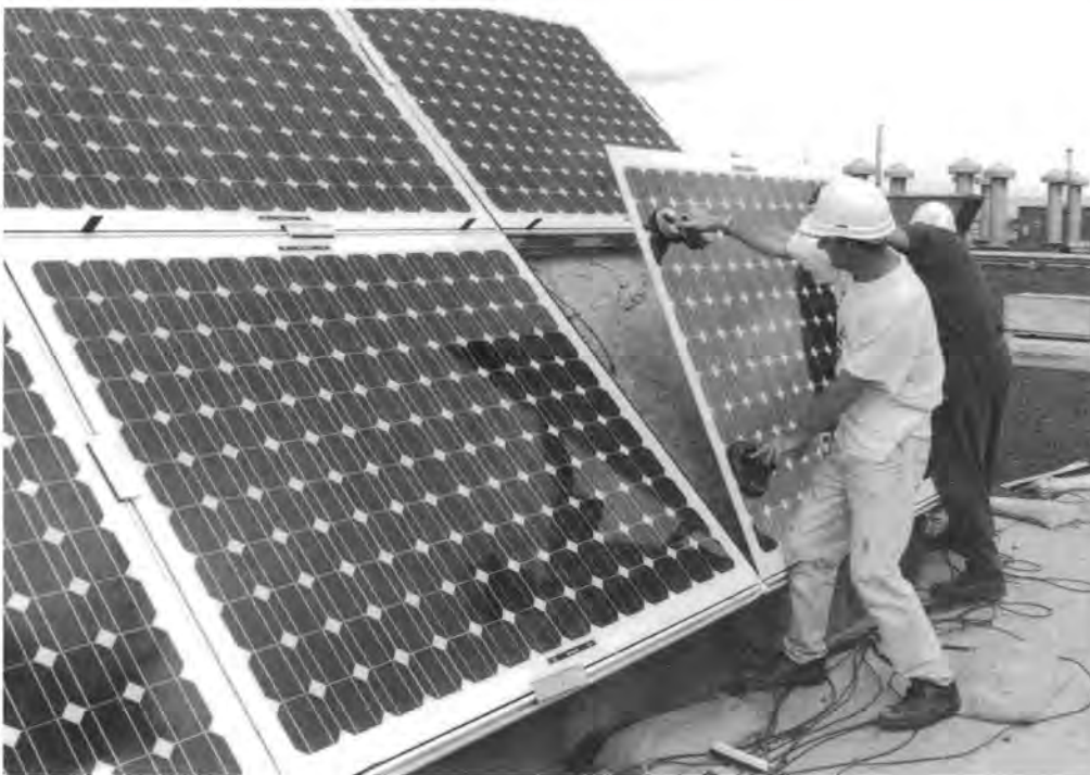
Installing photovoltaic panels on the roof of Ford's Bridgend engine plant
