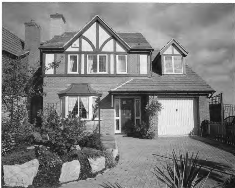
A perfect '10' for this Westbury house in Milton Keynes
