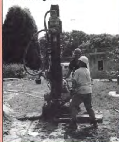
Drilling the boreholes in the school grounds
