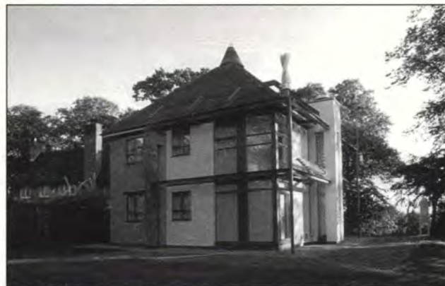
The Eco-Energy House, with passive ventilation stack, light pipes, and both PV and solar thermal collectors
