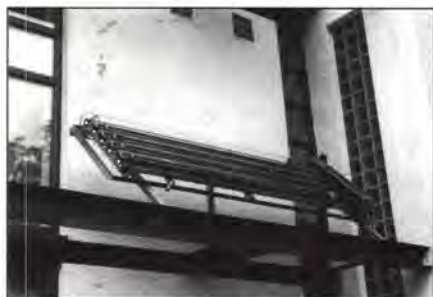
Evacuated tube solar hot water collectors fitted to the Eco-Energy House
