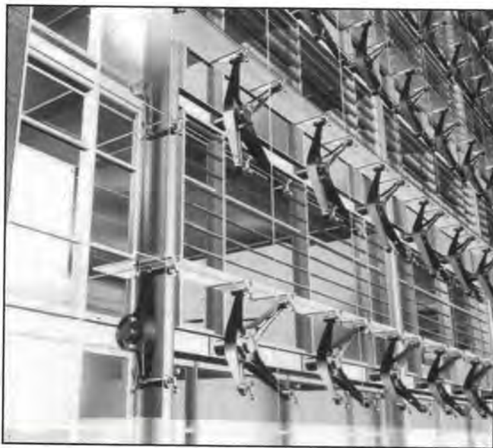
Louvres behind the outer glass screen wall will be automatically adjusted to either reflect or let in the sun's rays
