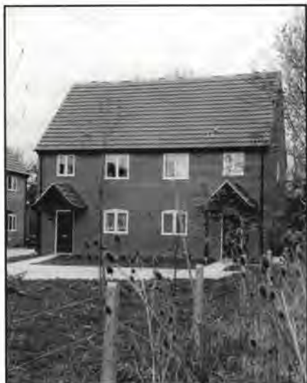
Hastoe Housing Association developed rural housing at Elsenham, Essex to test various water conservation measures and as a trial of environmental assessment using BREEAM.
