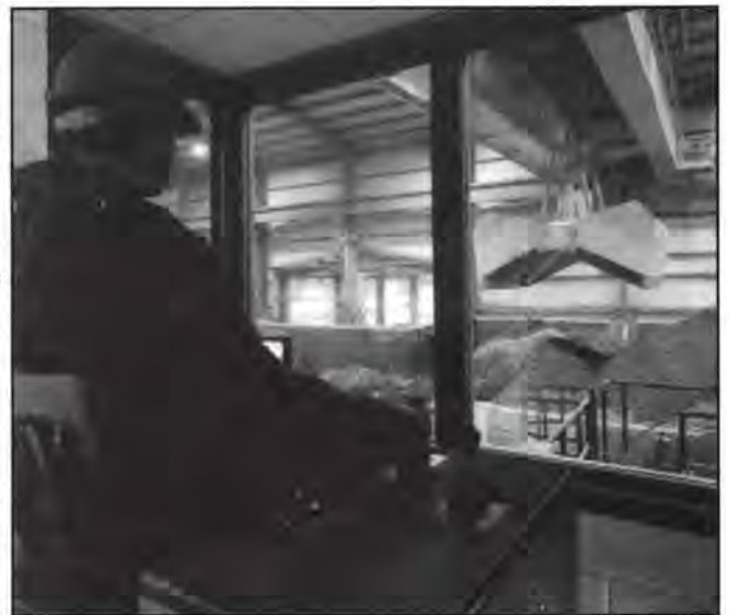
Fuel handling at the Westfield plant. Photo courtesy of Siemens Moore Process Automation, who supplied the process control system
