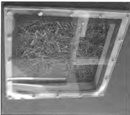
This page and opposite: Straw bale technology is incorporated into the external envelope of the new Faculty of the Built Environment Studies Building at the University of the West of England. Architect: White Design, engineer: Buro Happold. © Buro Happold/Adam Wilson
