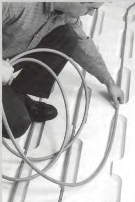
The pocketed polystyrene system simplifies the installation of heating pipe within a screeded floor and can also provide a base for an inexpensive timber floating floor.
