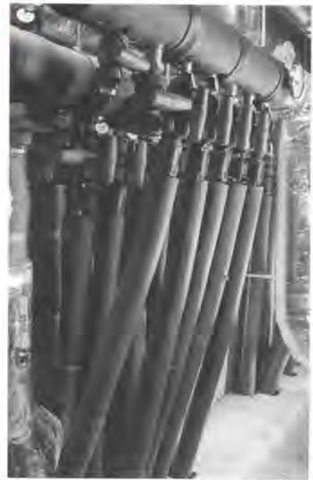
Energy efficiency in buildings – Applied Energy designed and installed a closed loop geothermal heating and cooling system for a major new commercial building in Croydon. The company calculated that a geothermal solution would give higher overall efficiencies than a conventional system. The picture shows geothermal loops entering the building onto a pipework header.
