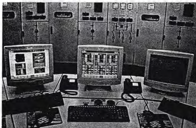
The control room
