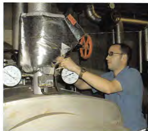
Adequate insulation on steam and condensate pipework reduces heat loss, resulting in improved efficiency of heat distribution
