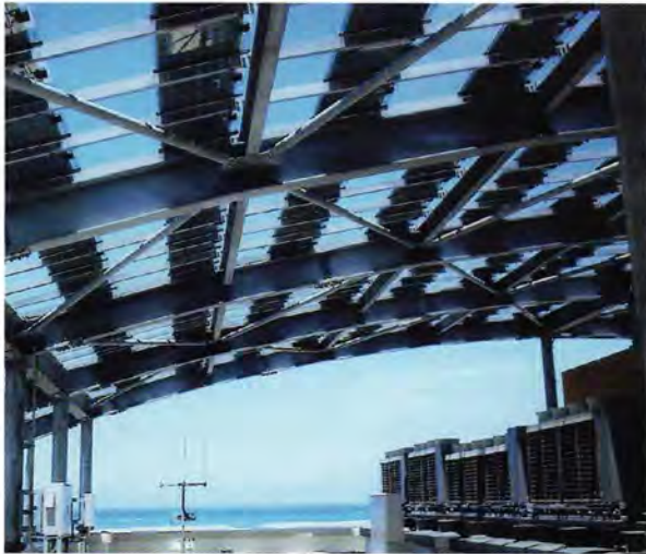
Horizontal louvres with integral solar cells
