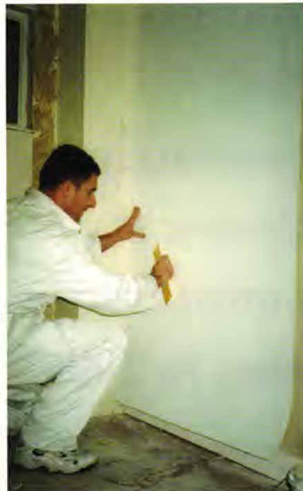
Applying insulated thermal lining – a step change in home insulation levels will be essential for meeting carbon dioxide reduction targets
