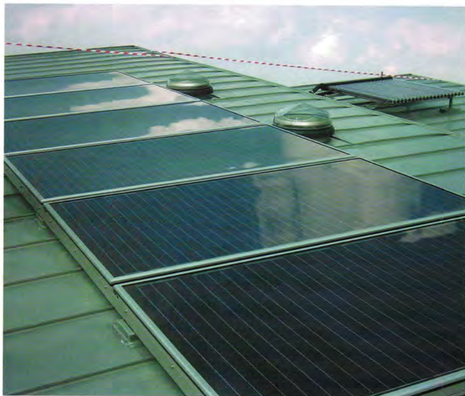
A 6.47 kWp PV array has been fitted on the south facing roof
