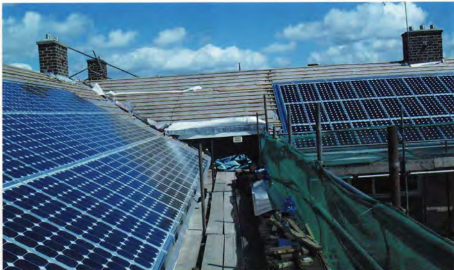
Site work included the addition of new boarding and a waterproof membrane beneath the PV modules
