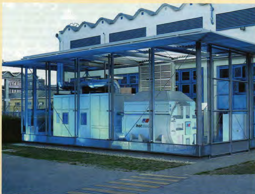
The first dual fuel 'HotModule' fuel cell unit from Germany's MTU CFC Solutions has gone into demonstration service at a CHP district heating plant in Berlin. The plant, which can run on natural gas and methanol, should demonstrate that the technology is not dependent on existing gas networks, but can also operate on liquid fuels, in this case derived from wastes generated in the city. The plant, based on technology from the US-based FuelCell Energy Inc, can produce 230 kW of electricity and 180 kW of heat at 400°C.
