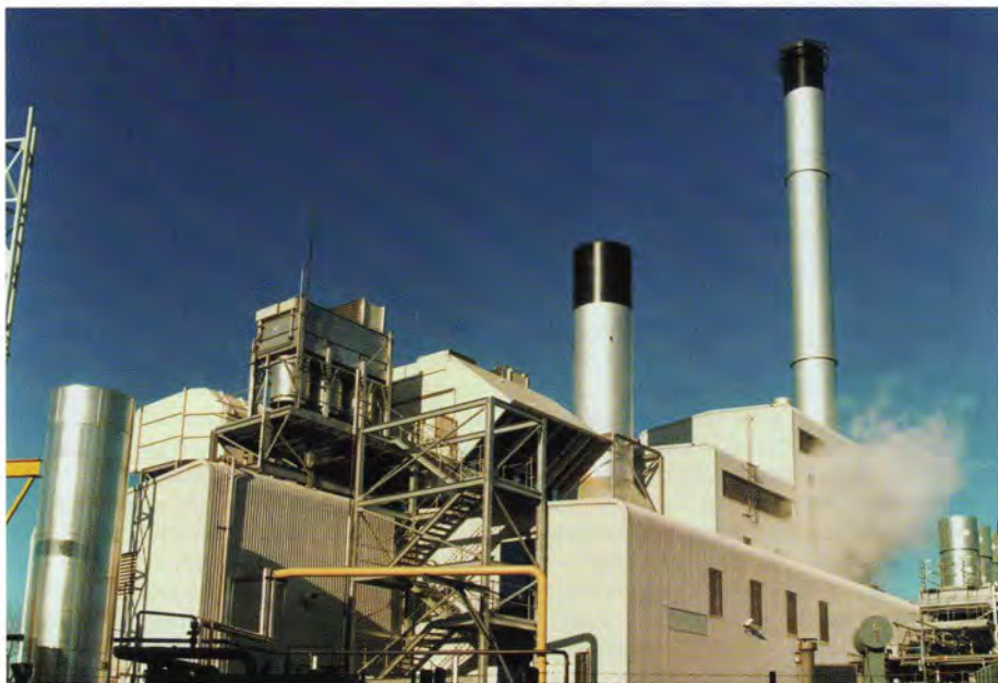
This CHP plant at British Sugar's Wissington factory near Downham Market in Norfolk, exports up to 50 MW to the national supply network from a 50 MW gas turbine and a 30 MW steam turbine
