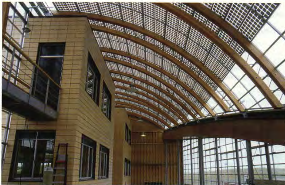
PV power in Europe – a new-build solar canopy
