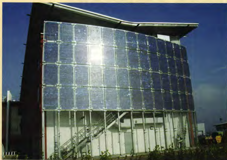
The Warwickshire County Council-owned Optima Innovation Centre at Elliot Park in Nuneaton is the largest PV installation in the West Midlands. In an impressive project that involves 105 kWp of solar capacity, BP PowerGlaz building-integrated laminate panels have been installed on the southern facing façade of the building, together with a Kalzip construction system housing 573 solar panels on either side of the East and West facing roof.
