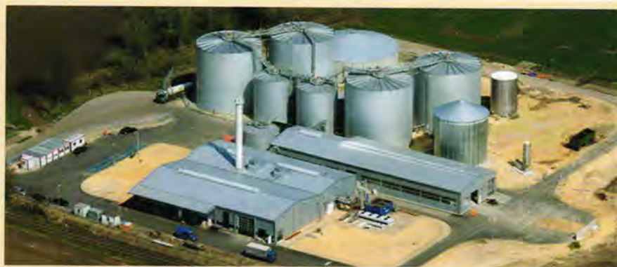
A new CHP biogas plant featuring GE Energy's Jenbacher gas engine systems has been commissioned in Northern Germany. One of Germany's largest biogas energy plants in terms of total output, the new facility will utilise corn and rye as biomass to power three cogeneration systems that will together generate 4.2 MW of electricity and 4.3 MW of thermal energy.
