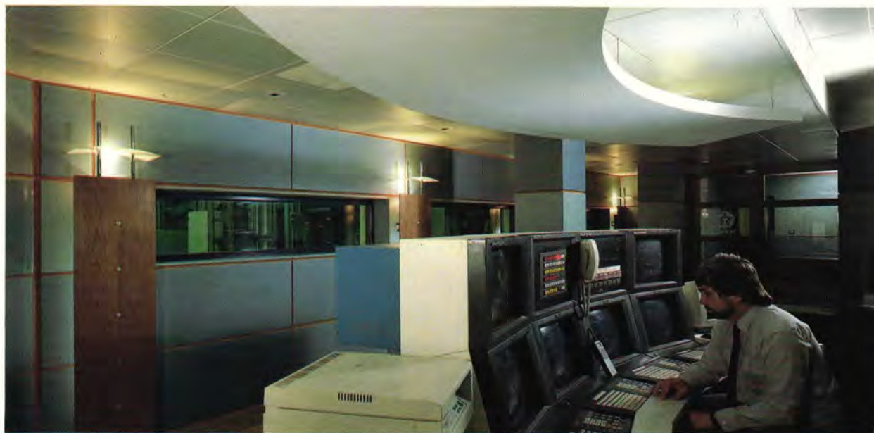
Texaco's new control room — designed to take the strain.
