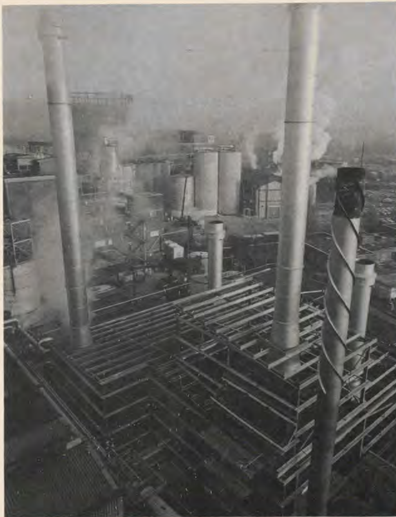
The CHP power house at Tunnel Refineries during construction.
