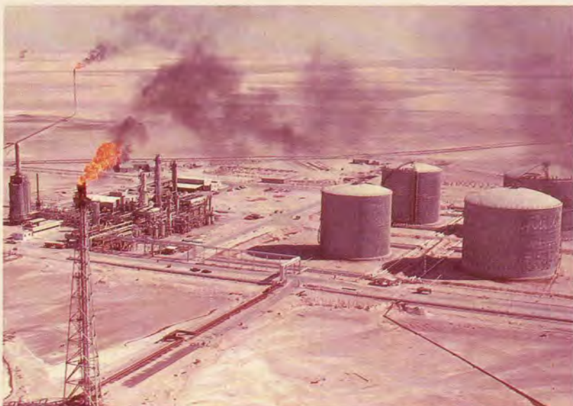
Umm Said plant
