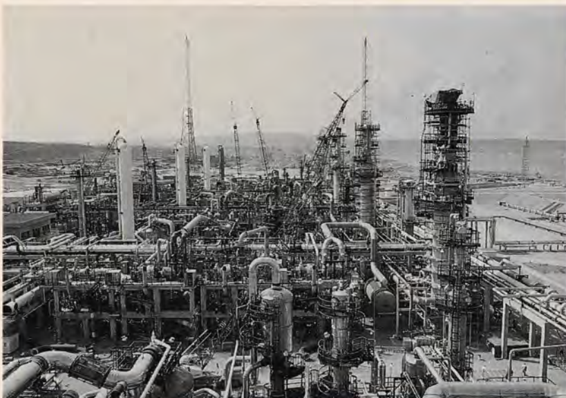
Liquefaction plant at Arzew.
