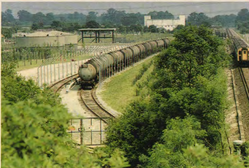
Kelt's Holybourne crude oil loading terminal.
