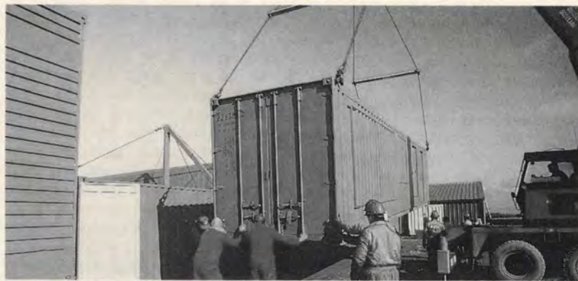
Ramco's PCU being unloaded at site.
