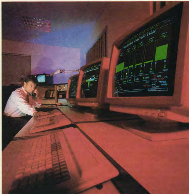
UKOP pipeline control system
