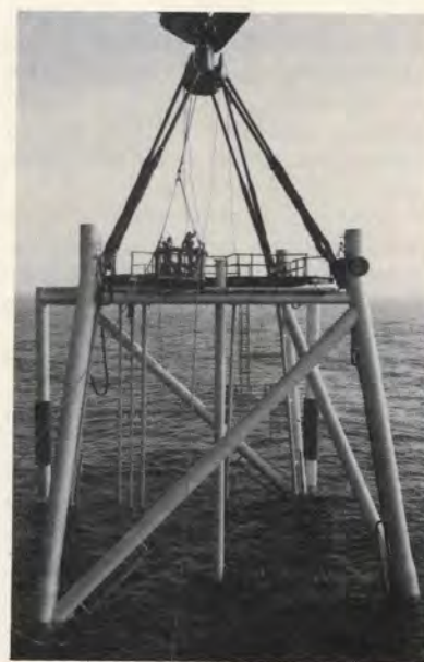
The Cohasset jacket being installed by the McDermott derrick barge.
