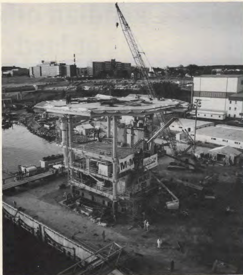
The Panuke deck awaiting its loadout. Photos courtesy of Nova Scotia Department of Natural Resources.
